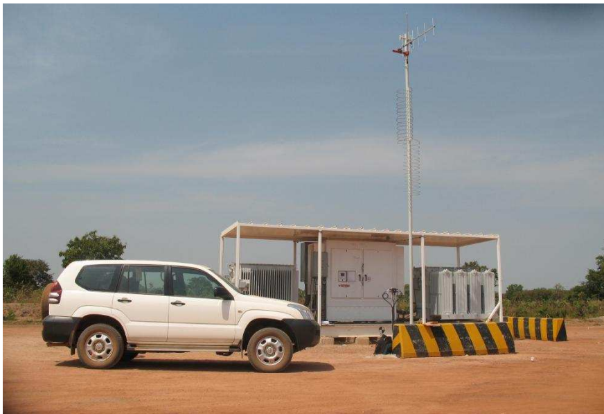
Skid Mounted Vector VII Drive with SCADA System and Transformers
